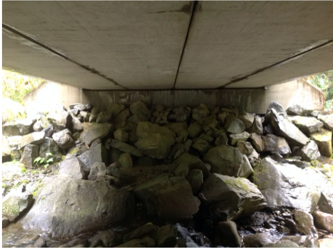
Left Bank Abutment when facing downstream
