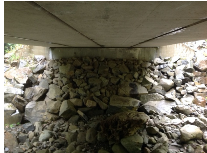
Right Bank Abutment when facing downstream
